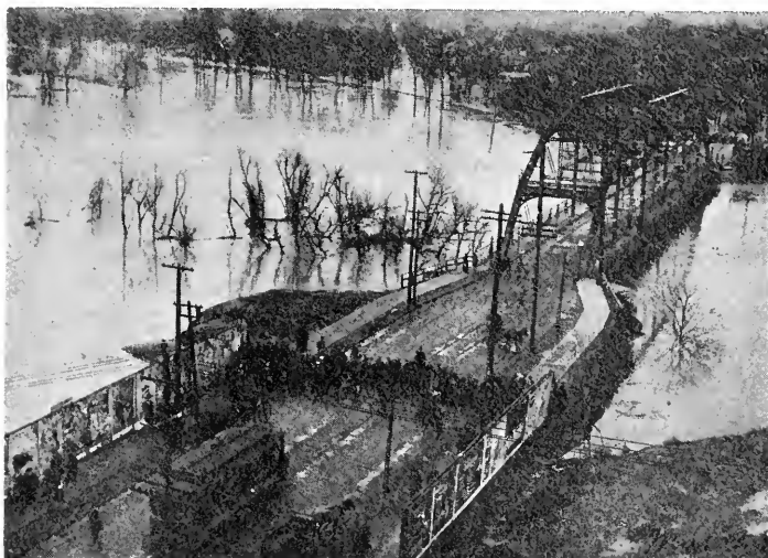
The New Steel Columbia Street Bridge of 1890
